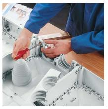
Adjust stepped grommet on the cable diameter.
